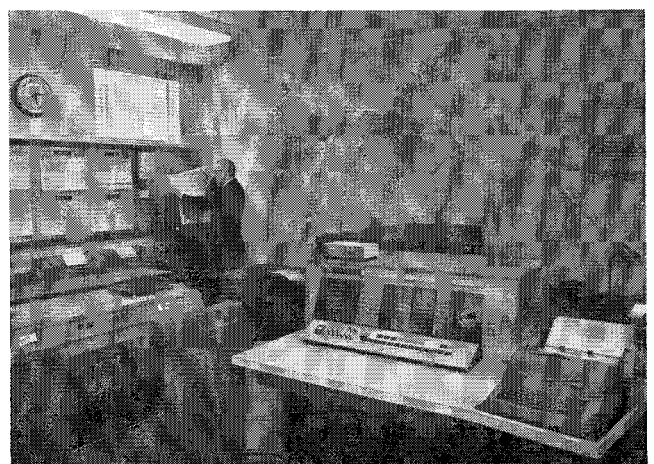
Fig. 2 General view of computer flight planning center showing IBM 1620 data processing system and weather data facsimile and teletype units.
